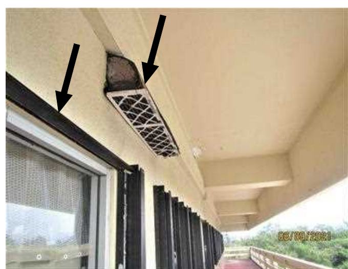
WINDOW SHUTTER HEAD AND EXHAUST HOOD
