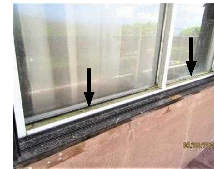
MILDEW ON WINDOW SILL WITH GREEN ALGAE (TYP. - 20ea.).
