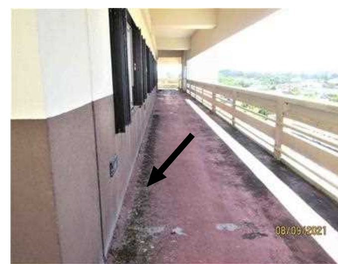
BIRD DROPPINGS FROM SHUTTER HEAD OR BEAM LEDGES LIGHT TO HEAVY INFESTED NARROW TO EXTRA WIDE AREAS.
