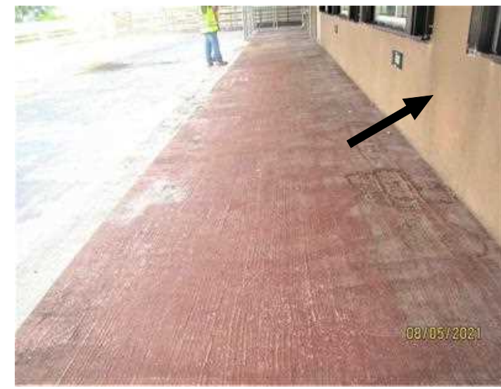
DETERIORATED WALL PAINT WITH STAINS & MILDEW (5100 sf).
