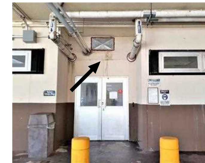
4e PHOTO S-1.2 | S-1.2.A STAINED WALL PAINT (±104 Sf).
