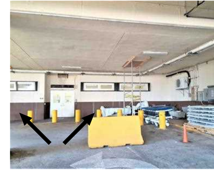
4e PHOTO S-1.2 | S-1.2.A STAINED WALL PAINT (±104 Sf).
