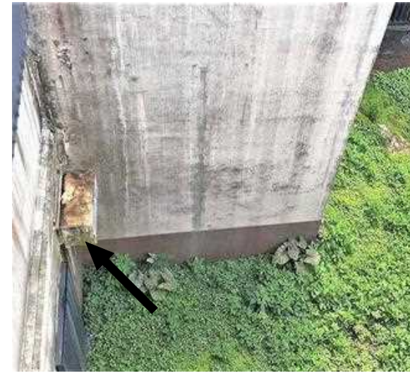
DETERIORATED WALL MOUNTED EXHAUST HOOD.
